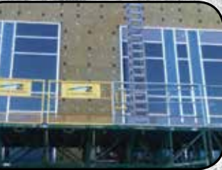
Behind cladding over steel stud walls
