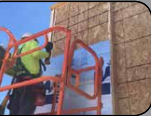
Behind cladding over wood stud walls
