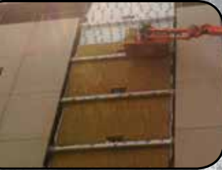
Behind cladding over concrete block walls
