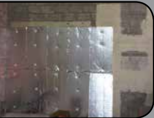
Interior walls on concrete block
